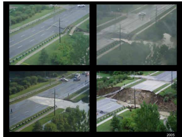
Fig. 13.3. Four views of a washed-out section of a major arterial roadway in Toronto after heavy rain and flooding of the Don River followed Hurricane Katrina, which was downgraded to a tropical storm when it hit Toronto on August 29, 2005. Photo-collage by Carmela Liggio and Nina-Marie Lister, 2005.
